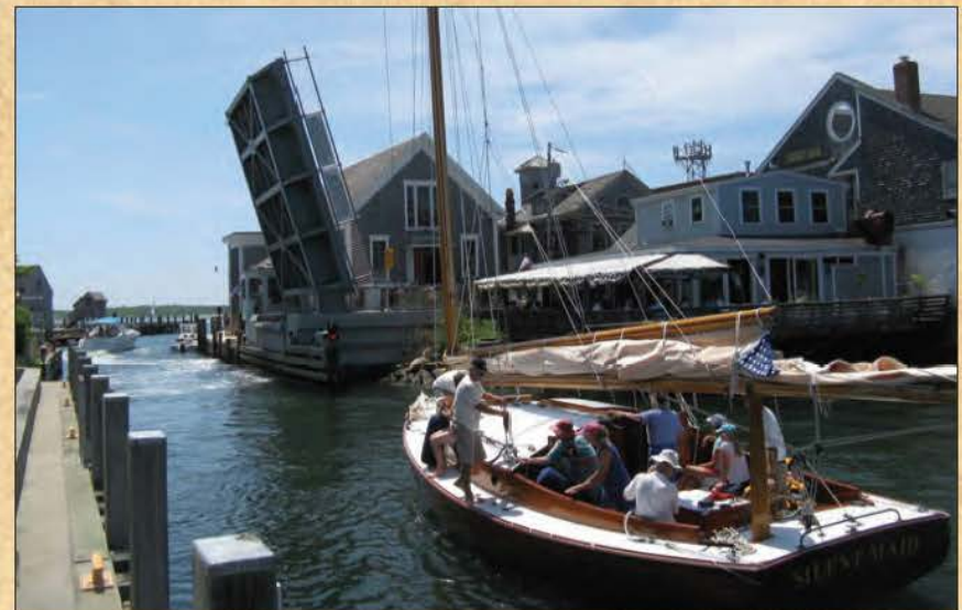
Eel Pond Bridge is raised on the hour and the half hour when a boat captain radios the Bridge Tender and requests passage into or out of Eel Pond.
