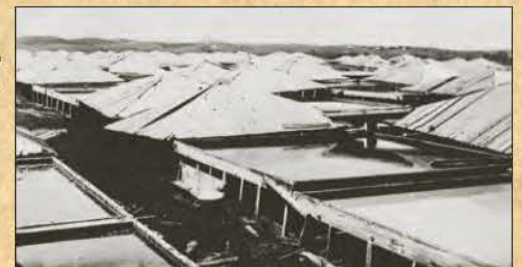
The evaporation vats had covers that were closed during rainy weather.
