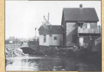
The original stone bridge A temporary, wooden pedestrian bridge was then put in place until the present-day drawbridge was built.
