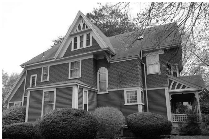
Watson house side view showing Queen Anne style asymmetrical window placement, varied textures of clapboards, shingles, and half-timbering. Photo by Susan Fletcher Witzell.
