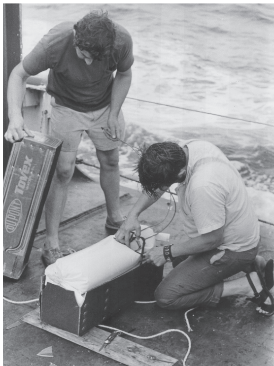
Tom Stetson and Donald Koelsch aboard Chain off the mouth of the Amazon River in June 1975. Koelsch was inserting a half pound block of TNT in a box containing two 60 lb. bags of TOVEX, an explosive gelatin. The corners were cut off so the boxes would sink when they went overboard. The TNT was used to detonate the TOVEX.
