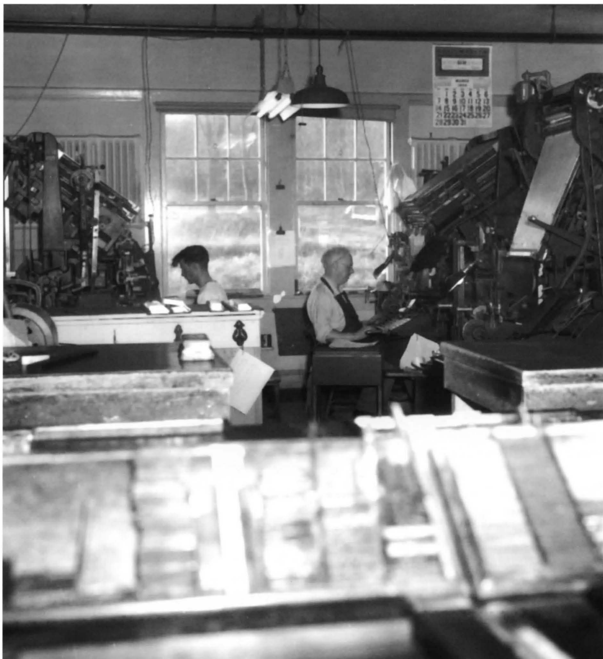
Linotype operators set reporter and ad copy into type for the next issue. Outside the windows are the railroad tracks and the edge of the woods leading up to Highfield Hall. In the foreground are banks of large type used in headlines.
