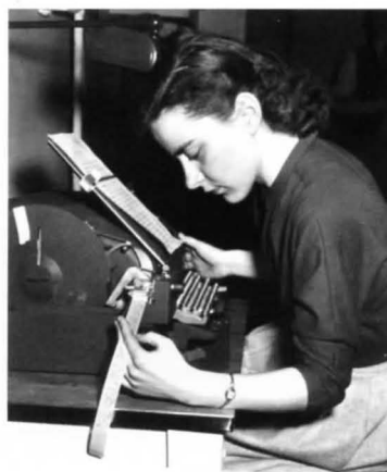
Vivian Hodgkins checks perforated type for the teletypesetter.
