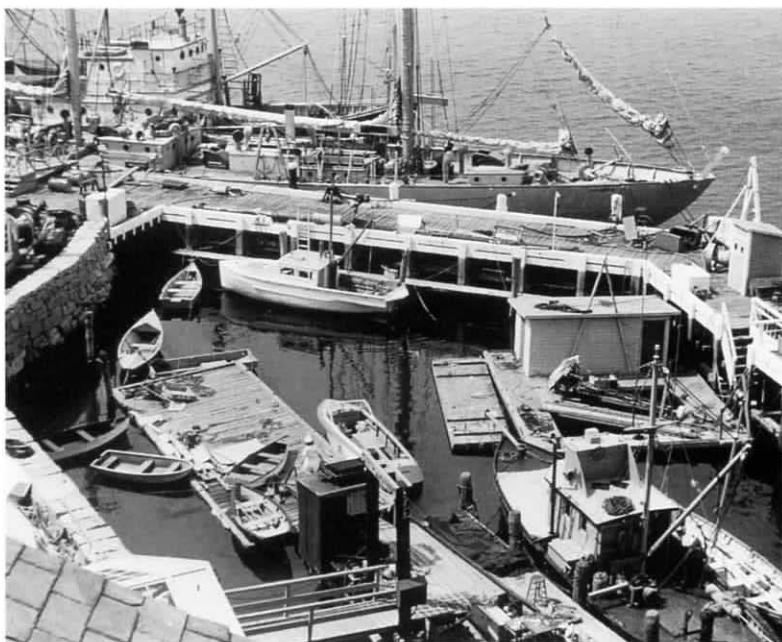
Atlantis moored starboard-side-to at the Woods Hole Oceanographic Institution dock, ca. 1945. Her gallows frame for deep-sea anchoring juts out from the bow toward those "derricks and little shacks along the dock edge" described in Olcott Gates' letter. Small boat basin in foreground. Photo by Paul Ferris Smith.
