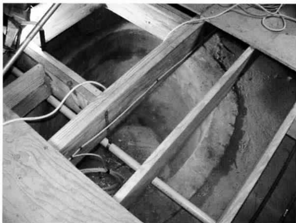
Original cistern in the cellar where run-off rainwater was collected for household use. Photo by E. Graham Ward.
