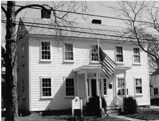
Front view of 16 Main St. under restoration. Sign identifying the house as the birthplace of Katharine Lee Bates stands to the left of the front door. Photo by Janet Chalmers.
