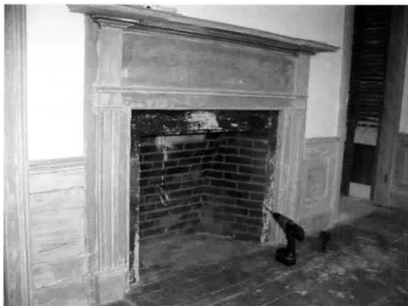
Upstairs Federal style mantel surrounding the fireplace. Most of the non-original green paint has been removed by hand sanding. Photo by E. Graham Ward.
