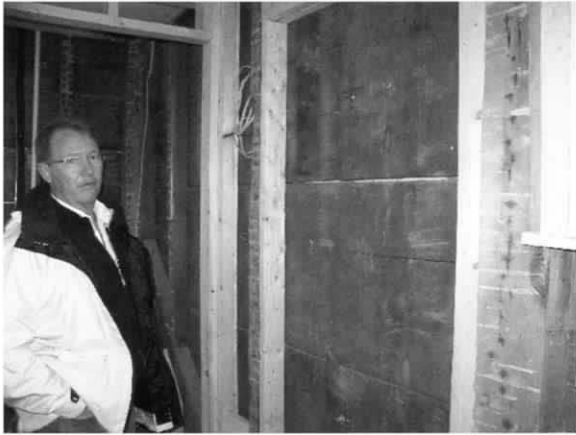
Restorer David Newton points out the original wide boards used in the construction of the house. Photo by E. Graham Ward.
