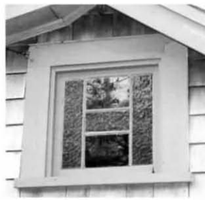
Outdoor view of frosted glass H window on Ward's Hodgson cottage. Photo by Janet Chalmers.
