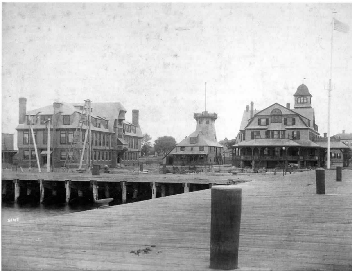
U.S. Fish Commission buildings in Woods Hole, 1890. Fisheries laboratory on the left, administration and residence building with its adjacent flag pole on the right. The time ball is on top of the shingled water tower in the middle. Photo by Baldwin Coolidge, No. 5147. Courtesy WHHC.
